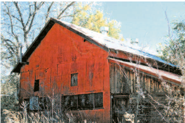
Former Mayor John Calkins' barn was used as the Village Maintenance Department in the 1950s.
