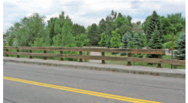
Existing Timber Railing
